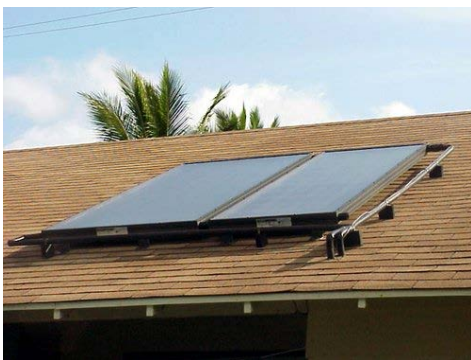
Figure A-1. Glazed flat-plate collector. Photo by Christopher Drake, NREL/PIX 09188
