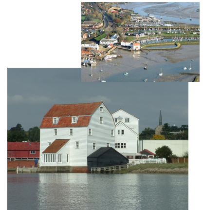
Figure 14.2. Woodbridge tide-pool and tide-mill. Photos kindly provided by Ted Evans.
