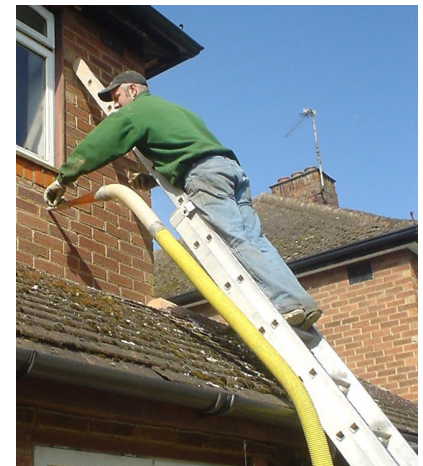
Figure 21.5. Cavity-wall insulation going in.
