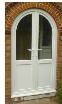
Figure 21.6. A new front door.
