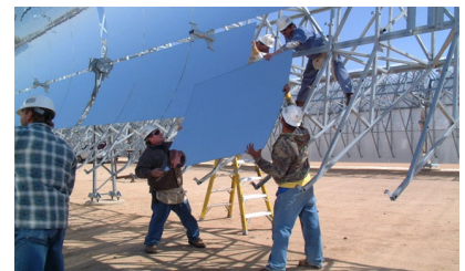
Figure 25.4. Andasol – a “100 MW” solar power station under construction in Spain. Excess thermal energy produced during the day will be stored in liquid salt tanks for up to seven hours, allowing a continuous and stable supply of electric power to the grid. The power station is predicted to produce 350 GWh per year (40 MW). The parabolic troughs occupy 400 hectares, so the power per unit land area will be 10 \text{ W/m}^2 . Upper photo: ABB. Lower photo: IEA SolarPACES.
