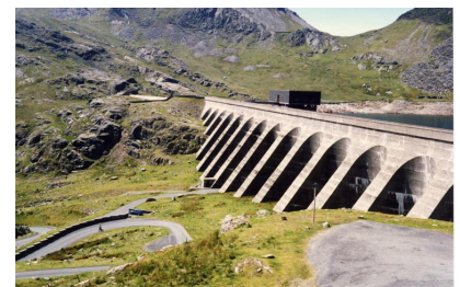
Figure 26.6. Llyn Stwlan, the upper reservoir of the Ffestiniog pumped storage scheme in north Wales. Energy stored: 1.3 GWh. Photo by Adrian Pingstone.
