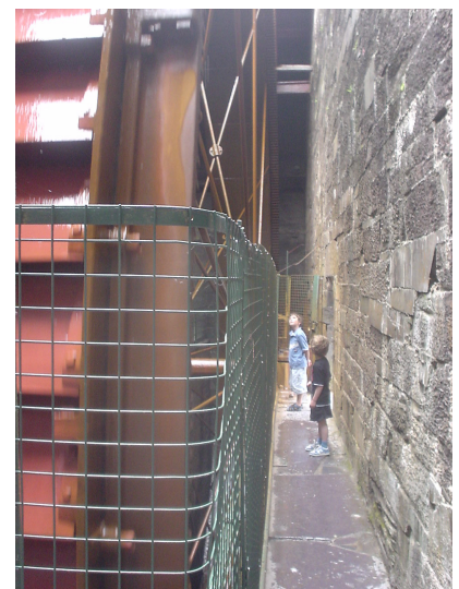
Figure 8.4. A 60 kW waterwheel.
