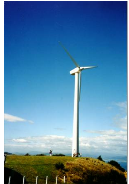
Figure B.3. The Brooklyn windmill above Wellington, New Zealand, with people providing a scale at the base. On a breezy day, this windmill was producing 60 kW, (1400 kWh per day). Photo by Philip Banks.
