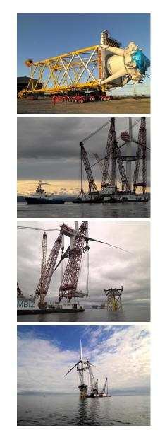
Figure 10.8. Construction of the Beatrice demonstrator deep offshore windfarm. Photos kindly provided by Talisman Energy (UK) Limited.
