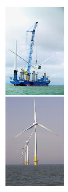
Figure 10.1. Kentish Flats – a shallow offshore wind farm. Each rotor has a diameter of 90 m centred on a hub height of 70 m. Each "3 MW" turbine weighs 500 tons, half of which is its foundation.
